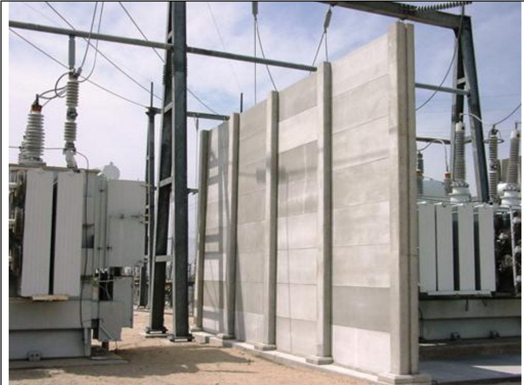
Installed modular refractory concrete firewall
